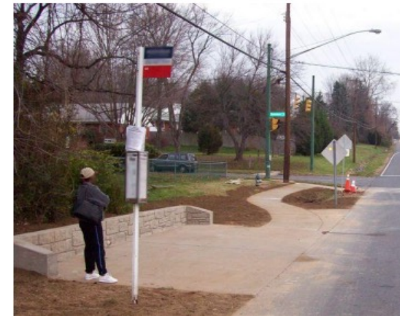
Bus stop landing pad
