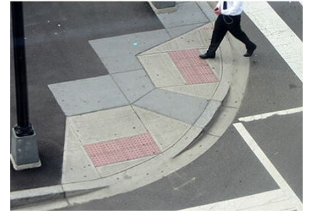
Accessible curb ramps
