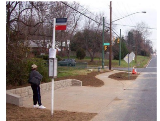
Bus stop landing pad
