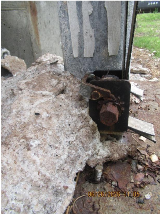
Southside – Bolts, Shackles, and Cables (See Drawing "Plan, Section & Details" – 2C)
