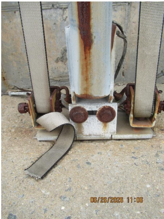
Eastside – Bolts, Shackles, and Cables (See Drawing "60' x 45' Anchor Bolt Layout" – 3C)
