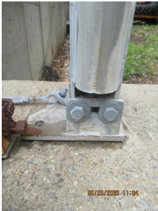
Westside – Bolts, Shackles, and Cables (See Drawing "60' x 45' Anchor Bolt Layout" – 4B)
