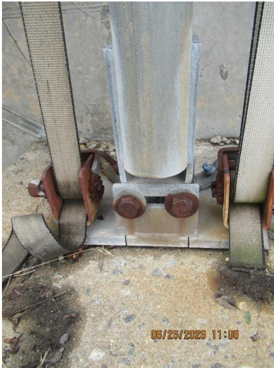
Eastside – Bolts, Shackles, and Cables (See Drawing "60' x 45' Anchor Bolt Layout" – 3C)
