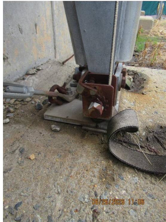
Eastside – Bolts, Shackles, and Cables (See Drawing "60' x 45' Anchor Bolt Layout" – 3C)
