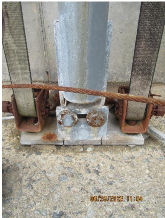
Westside – Bolts, Shackles, and Cables (See Drawing "60' x 45' Anchor Bolt Layout" – 3C)
