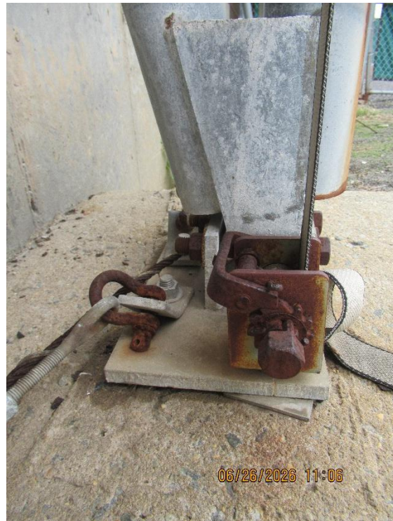
Eastside – Bolts, Shackles, and Cables (See Drawing "60' x 45' Anchor Bolt Layout" – 3C)
