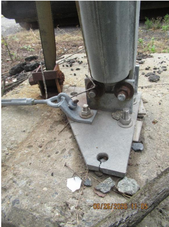
Eastside – Bolts, Shackles, and Cables (See Drawing "60' x 45' Anchor Bolt Layout" – 1A)
