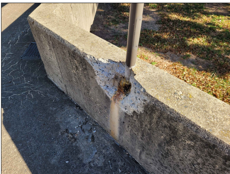
SPALL ON PARAPET WALL AT RAMP
