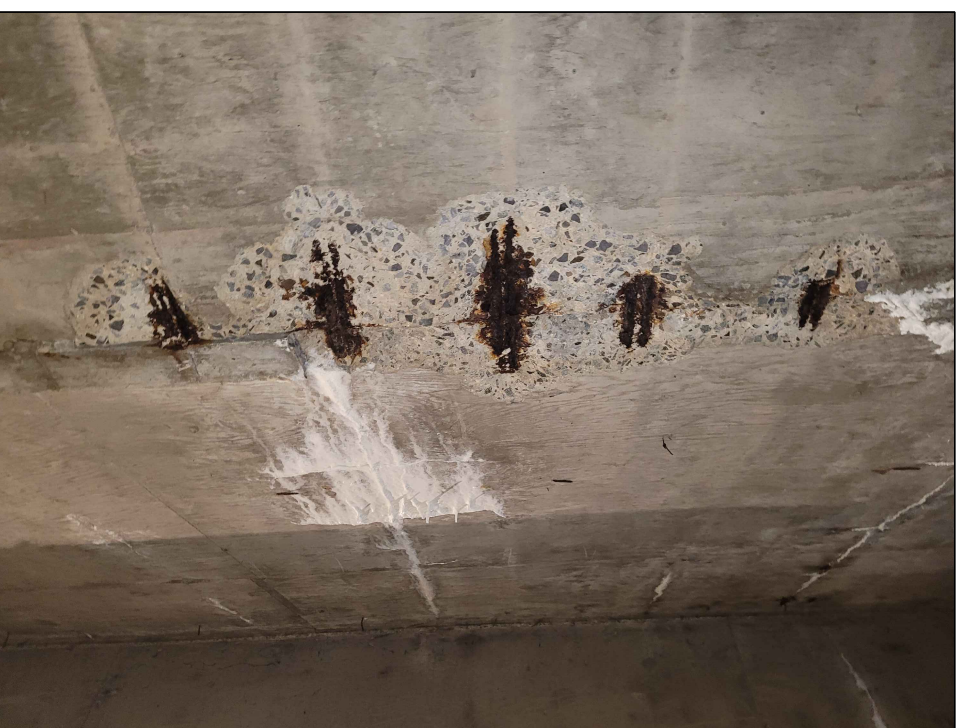
SPALL WITH EXPOSED REBAR AT UNDERSIDE OF STAIRS
