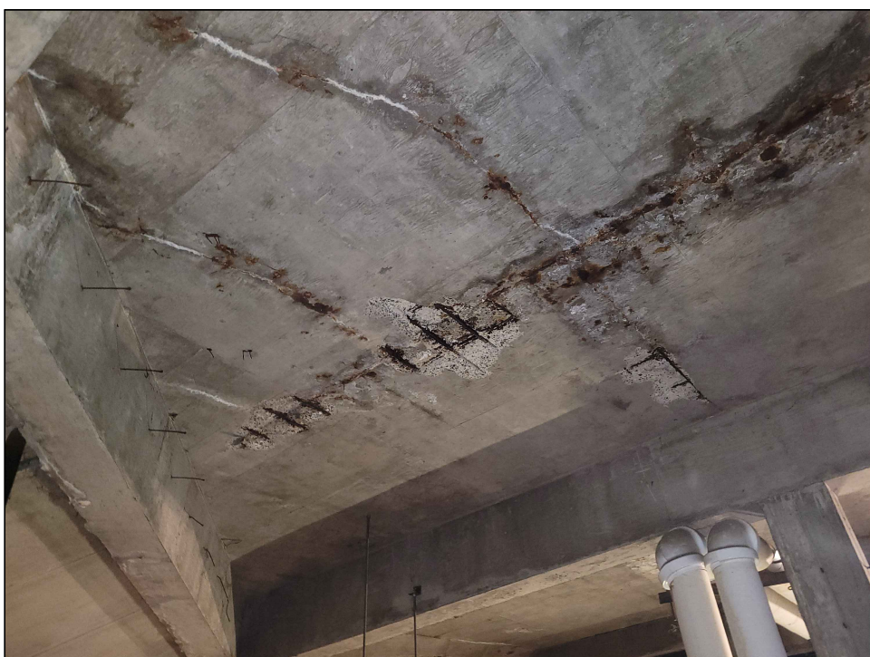
SPALL WITH EXPOSED REBAR AT UNDERSIDE OF PLAZA
