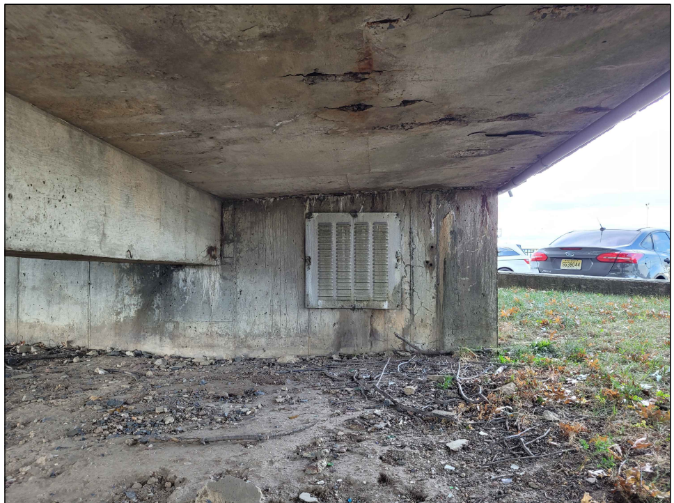
EXISTING WALL EXHIBITS CRACK/ EFFLORESCENCE/STAINING
