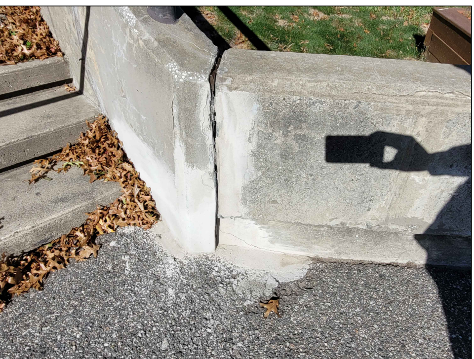
DELAMINATION AND JOINT MATERIAL FAILURE
