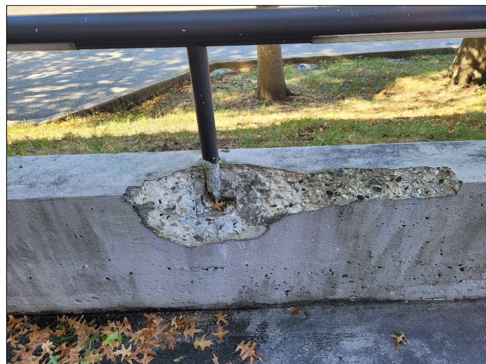
TYPICAL SPALL AT PARAPET WALL RAMP STRUCTURE
