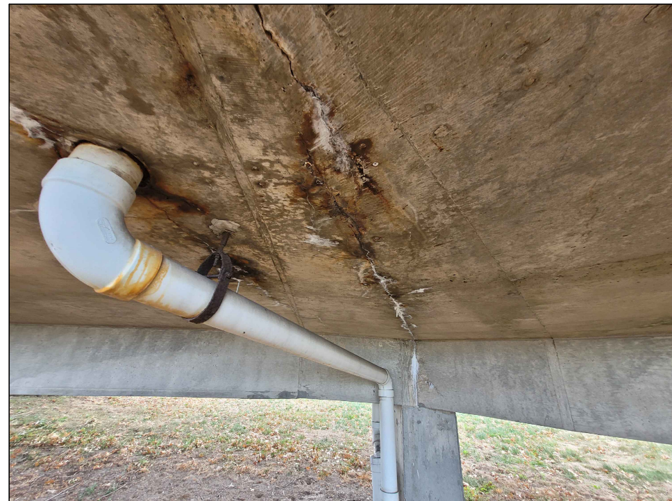
RAMP EXHIBITS CRACKS/LEAKS WITH EFFLORESCENCE (UNDERSIDE RAMP)
