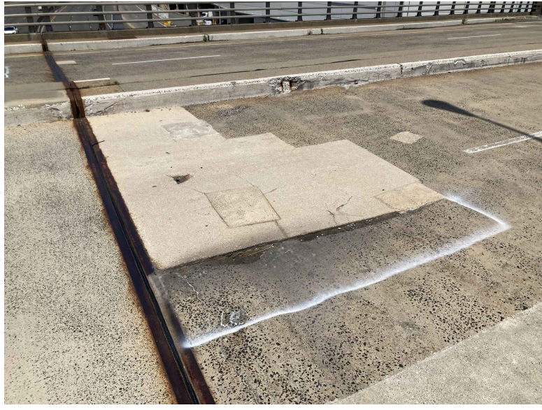
REPAIR DEEP SPALLS AT SPAN 2 IN EASTBOUND LANES NEAR PIER DECK JOINT
