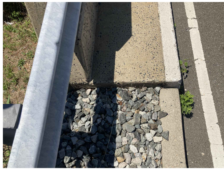
REBUILD THE SETTLED SOUTHWEST AND SOUTHEAST APPROACH CURBS
