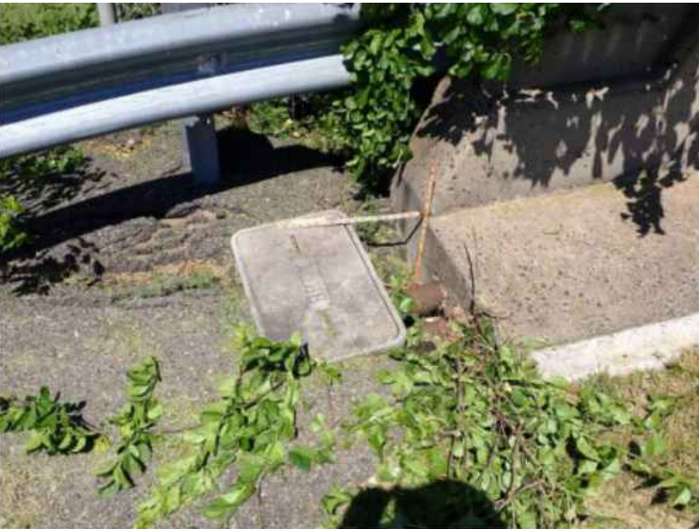
FILL AREA AROUND UTILITY BOX AT NORTHWEST APPROACH
