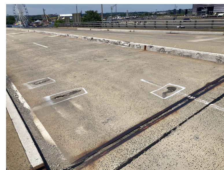
REPLACE SETTLED/TORN JOINT MATERIAL AT BOTH ABUTMENT DECK JOINTS
