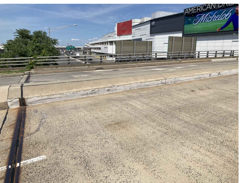
REPAIR THE SPALLS IN THE TOP OF DECK AND ABUTMENT DECK JOINT HEADERS
