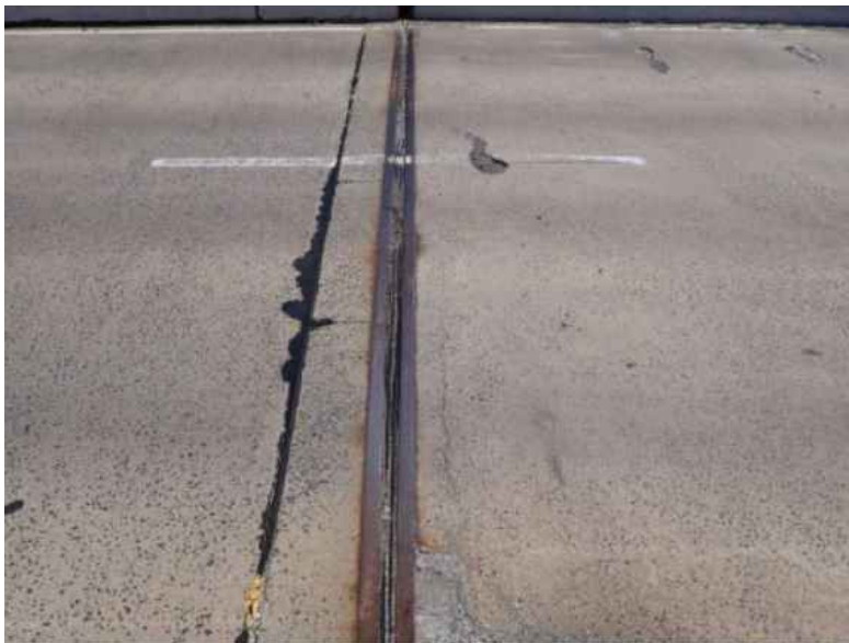
SEAL THE CRACK IN TOP OF DECK
