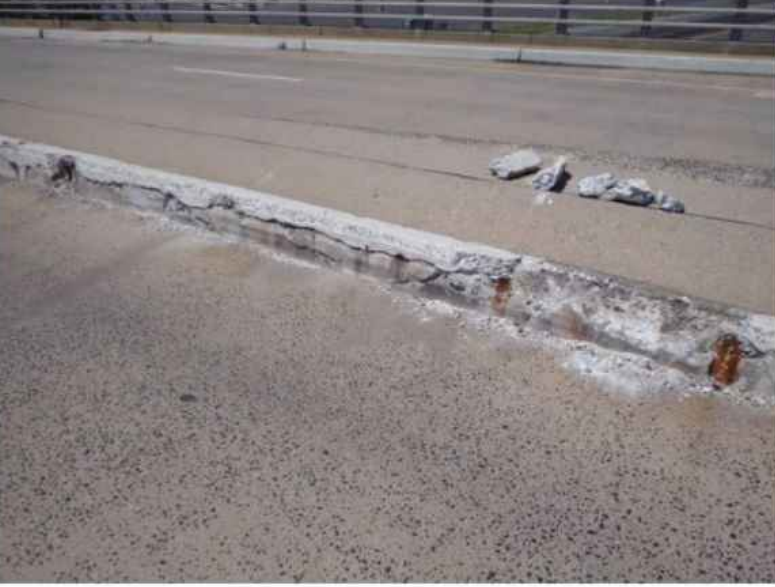
REPAIR SPALLED CURBS
