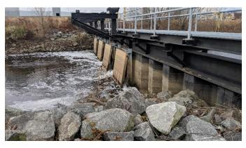
Figure 24 West Riser Tide Gate Downstream Face
