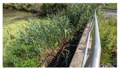
Figure 16 – Upstream View of Vegetation and Debris at Rutherford Tide Gate
