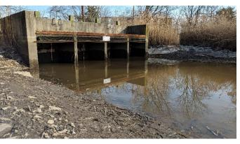
Figure 23 East Riser Tide Gate Downstream Face
