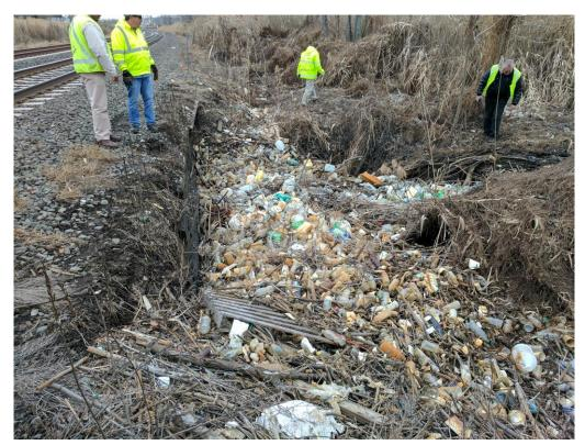
Figure 11 - Culvert with Floatables under NJ Transit Tracks
