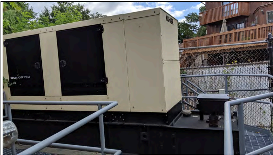
Figure 2: View of emergency generator
